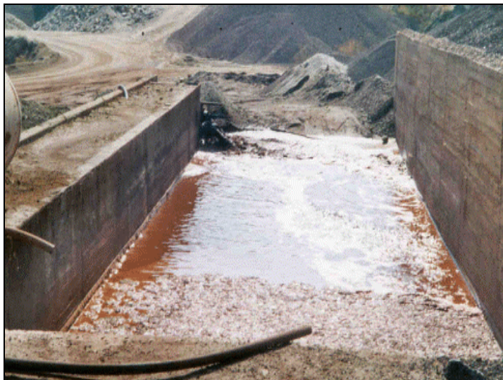
Figure 3.49: Dewatering of tailings in concrete basins [110, IGME, 2002]
