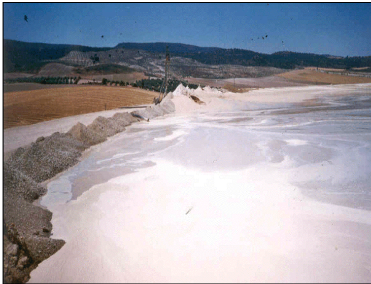
Figure 3.57: Old strontium TMF with tailings in structural zone [110, IGME, 2002]
