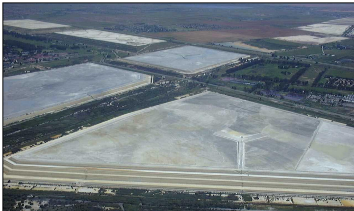
Figure 2.31: Tailings pond on flat land (Courtesy of AngloGold, South African Division)
