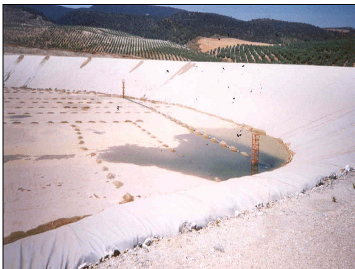
Figure 3.58: New strontium TMF with a synthetic liner and decant towers [110, IGME, 2002]
