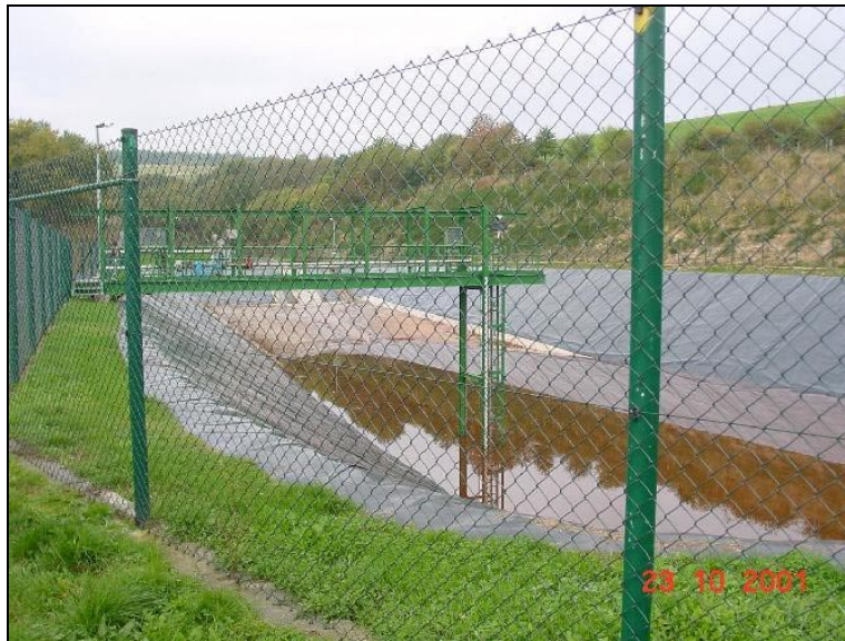
Figure 3.74: Water retention basin of German potash mine
