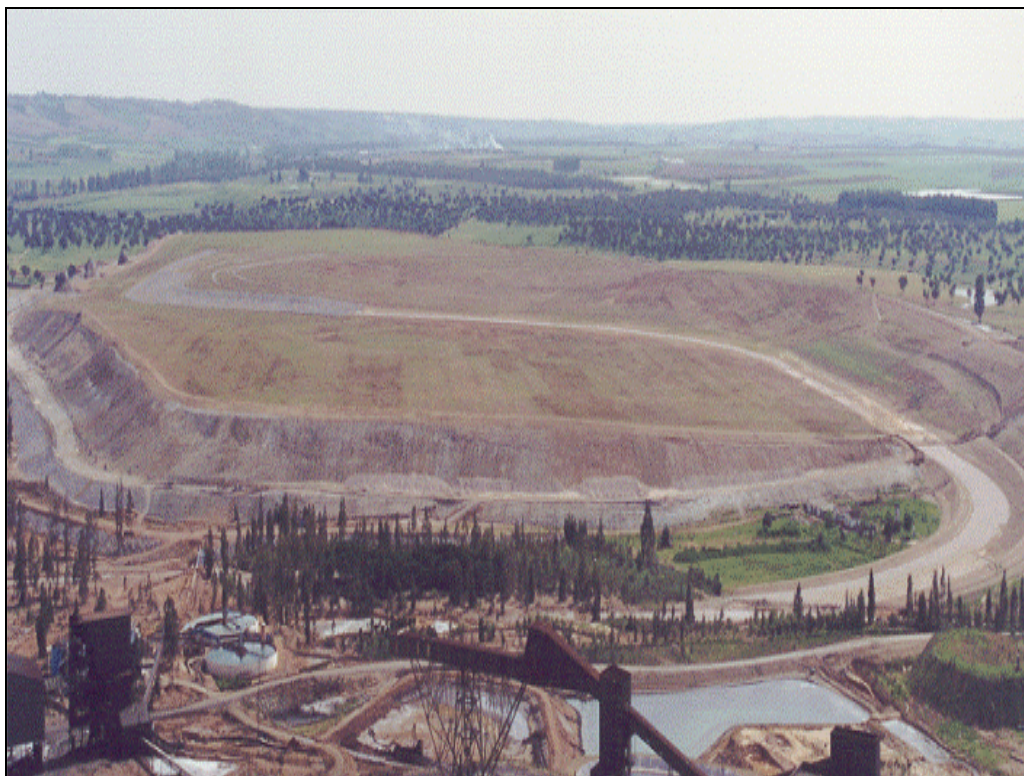
Figure 4.6: Collection and discharge channel at closed Apirsa tailings pond
