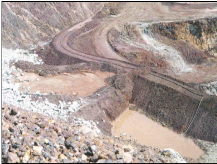
Figure 3.48: Dewatering of barytes tailings in the pit [110, IGME, 2002]
